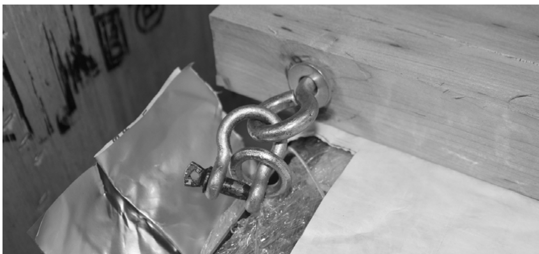
Figure 4-14. Attaching Eye-bolts to Spreader Bar
