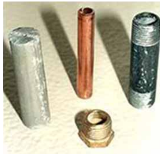
Treated Water Circuit
