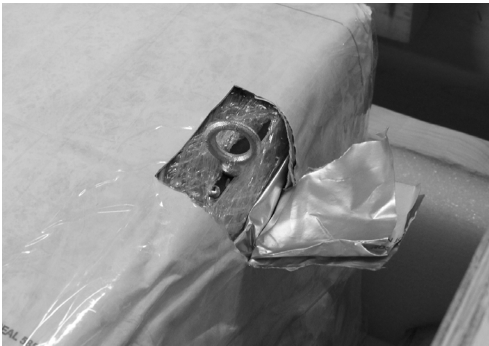
Figure 4-12. Installation of Eye-bolts
